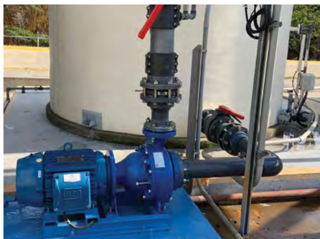
Finish Thompson UC Series mag drive pumps provide safe, reliable fluid transfer for odor control systems applications.
