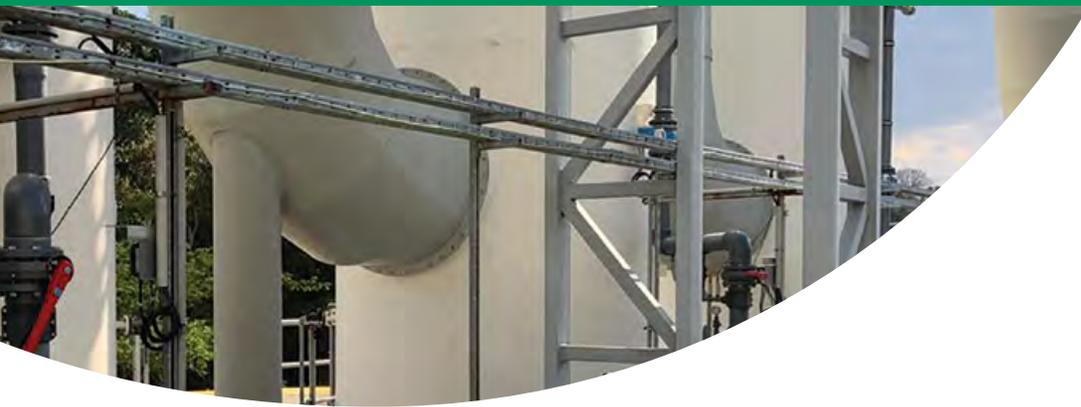
Once the Finish Thompson UC pumps were installed, the issues ceased. "Their UC pumps are almost two years old now and have experienced no problems," notes Gilberto. Switching from the sealed pump technology to magnetic coupling eliminated the issues with worn seals and the inevitable leaks they caused.
