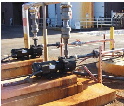
IMAGE 1: Self-priming pumps (Image courtesy of Finish Thompson)
