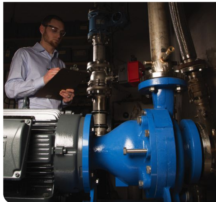
FIGURE 1: A lab technician is checking pump performance. This ULTRAChem pump is used for pumping a variety of caustic chemicals in an industrial lab. Courtesy Finish Thompson
